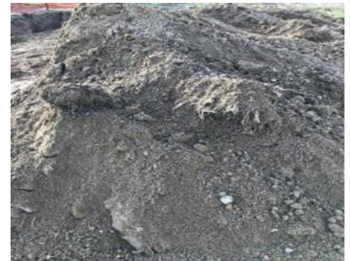
Spoil Pile - Type B Soil
